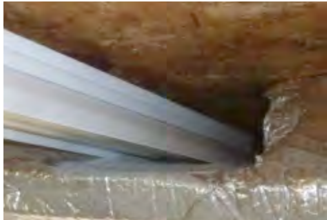
LED fixture just fits over the garage door.
