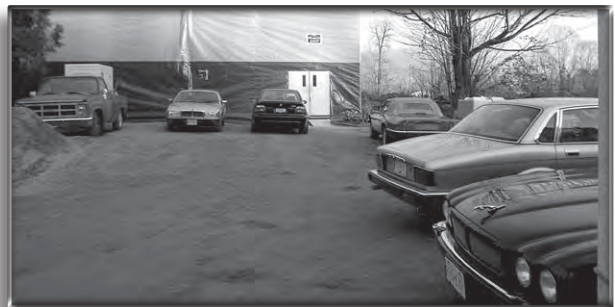
New car storage facility for the expanding Newby fleet
